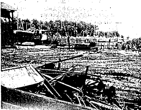
THE REMAINS OF THE BOATYARD FIRE.... A PILE OF SCRAP IRON.....
